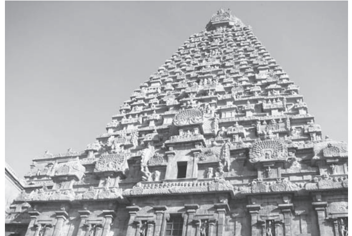
The Sri Brahdeswarar Temple was built by the great Chola king Raja Raja I in the 10th century.
