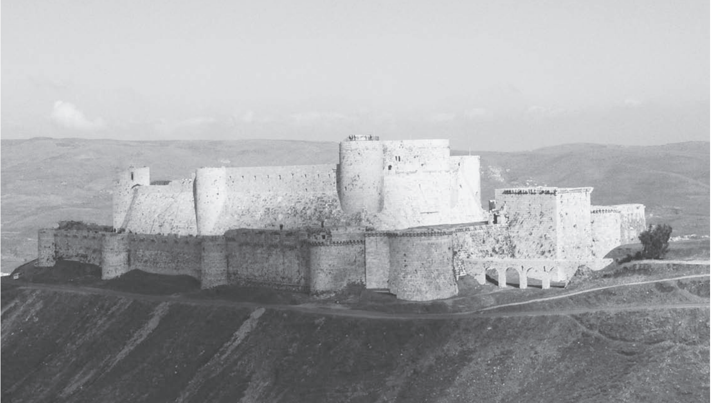
The Krak des Chevaliers, or knight's fortress, in Syria, built during the Crusades. Krak des Chevaliers was the headquarters of the Knights Hospitaller. It was expanded between 1150 and 1250; the fortress has outer walls 100 feet thick.
