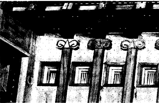
23. Detail of nave of the Jerusalem temple, from model by E. G. Howland, showing pilasters with "proto-Ionic" capitals after examples from Samaria and Megiddo, and windows with recessed frames
